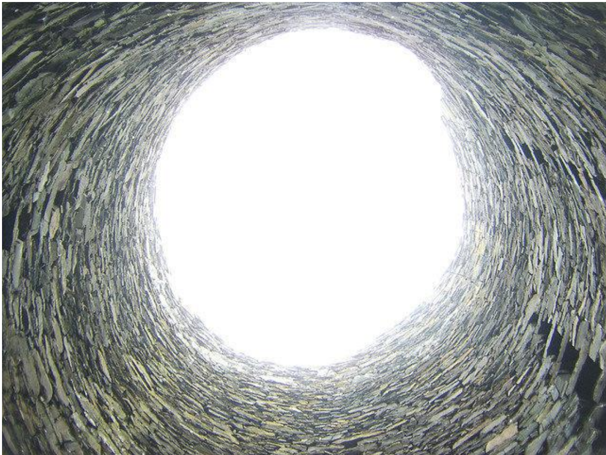
Figure 8 View looking up through the roofless broch at Mousa
