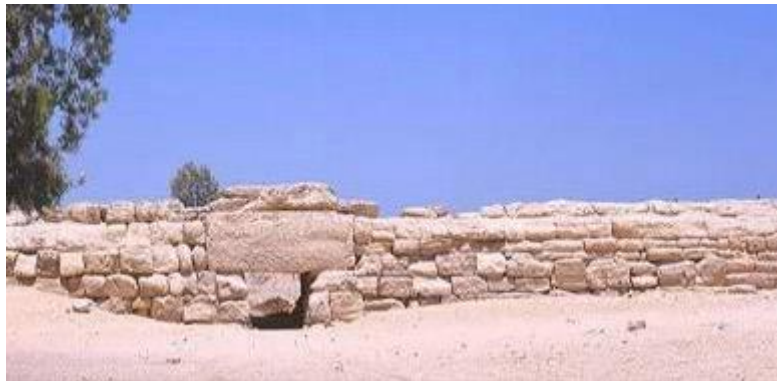
Figure 60 Wall of the Crow showing the Immense Stone Lintel above the passageway
